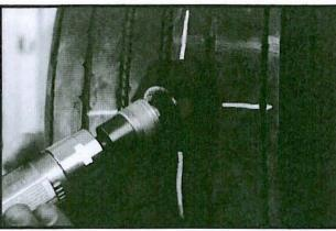
Clean the complete skived area and buffed perimeter on the inner liner with a soft wire brush mounted on a low rpm air buffer. The rotation of the brush makes it necessary to buff from the right side of the prepared surface to the left.
