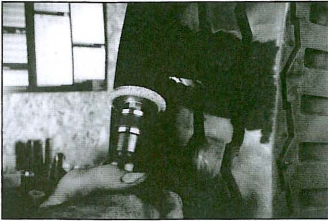
14 With the same rasp or an innerliner wheel (#RH-106), lightly buff a perimeter around the skive area approximately 1½" (40mm).
